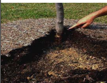
Mulch Depth too Deep
